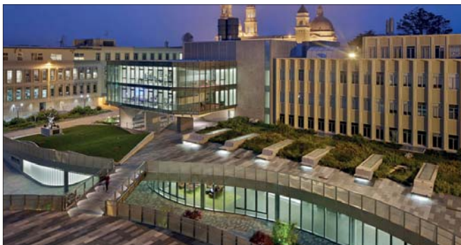
Harney Plaza Landscape, Center for Science and Innovation San Francisco Arkitekt: INTERSTICE/NBBJ
